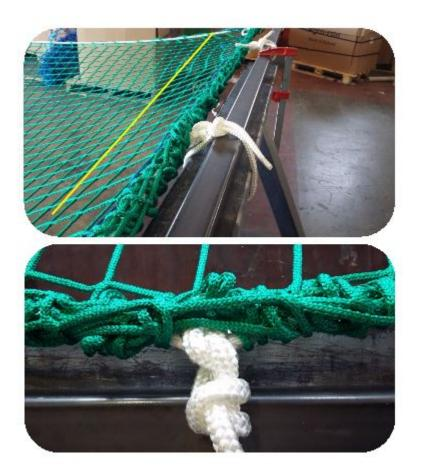
The meshes are parallel to the rolled (see blue rope acting as a reference) and the sag is not deformed.
