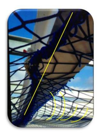
The border rope (and the rest of the rolled) has not an straight alignment, so the net has not been installed applying the same forces around the net and provoking the break in the overtensioned area because the net is not designed to absorb all the energy, being the border rope jointly with the main mesh the responsible of carrying out that aim.
