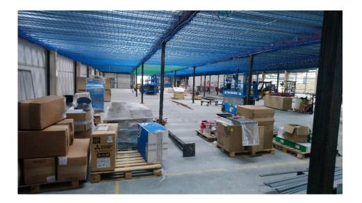
During the construction and as metal structure which is to be it has some risks to be sorted. For example **falls from workers** while the steed deck is being installed. Thus, we need safety nets for mezzanines. In that case we suggest to use of our safety nets EN 1263.1 type S A2 Q100 made in knotless polypropylene or in knotted polyamide.
