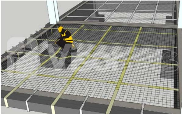
· the working platform nets will be fastened by their border rope by means of tie ropes or straps every 50 cm, whereby ropes or straps will have a minimum breaking strength of 30 kN. It is necessary to attach a minimum of 2 consecutive sides of the net to the supporting structure. The other/s side/s could be attached to the structure by means of clamping belts.
