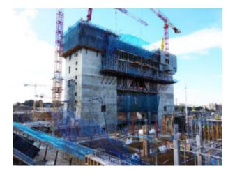
V-type nets are a system consisting of a safety net with a border rope attached to metal gallows by means of tying ropes. This way the fall of people and objects is limited from a maximum permitted height of 6 meters and recommended 3 meters.
